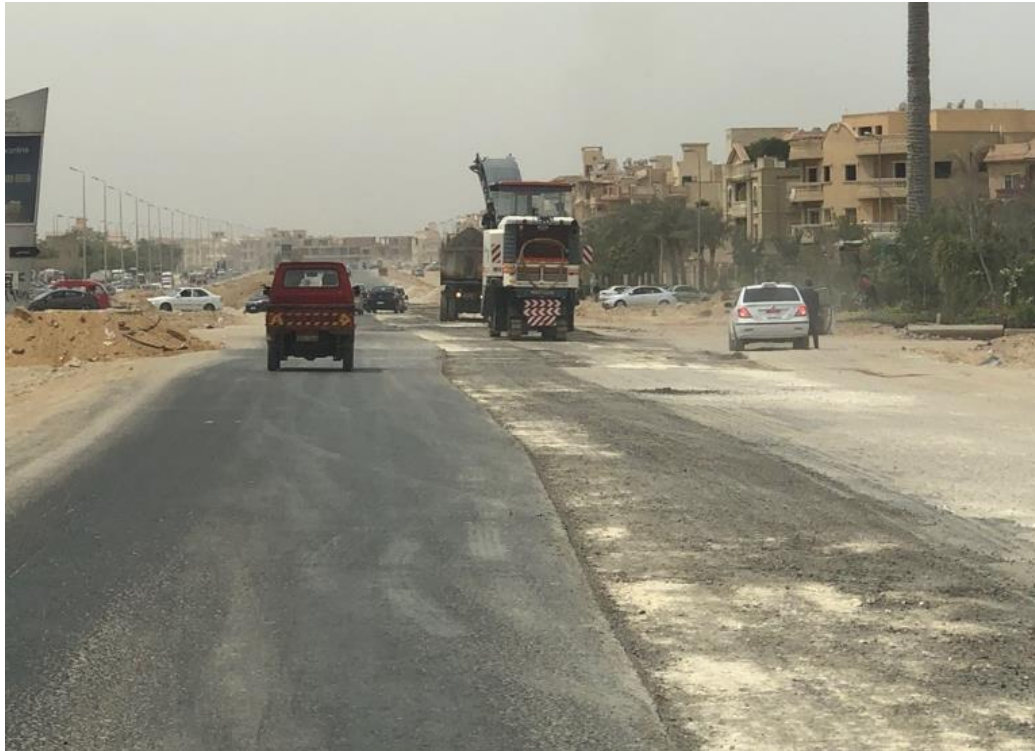
Figure 40: Paving North 90 Street in April 2018
