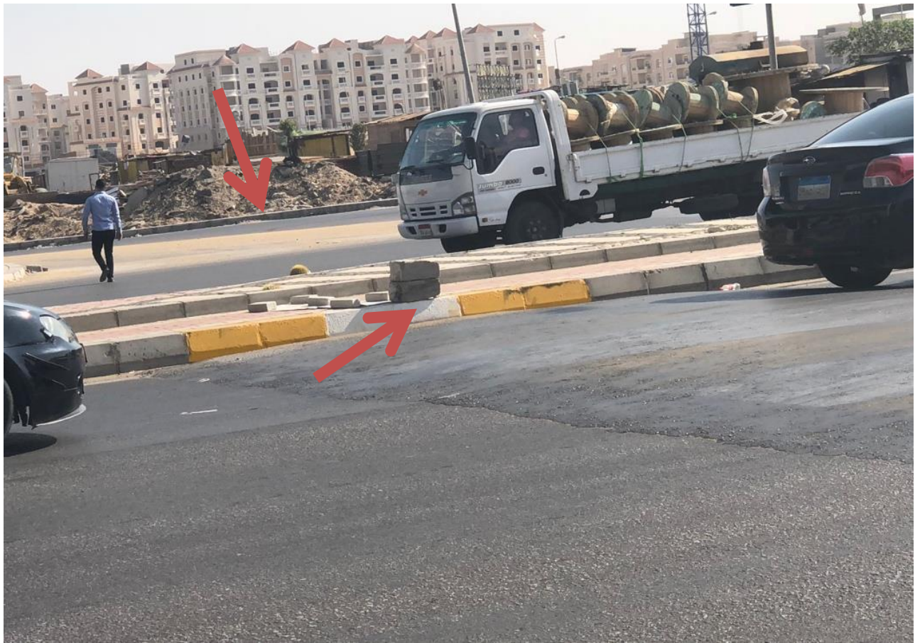
Figure 36: The wrongly used lacquer paint wears off quickly on the asphalt but not on the pavement sides where there is no friction
