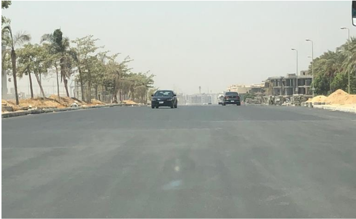
Figure 42: North 90 Street Newly Paved in August 2018
