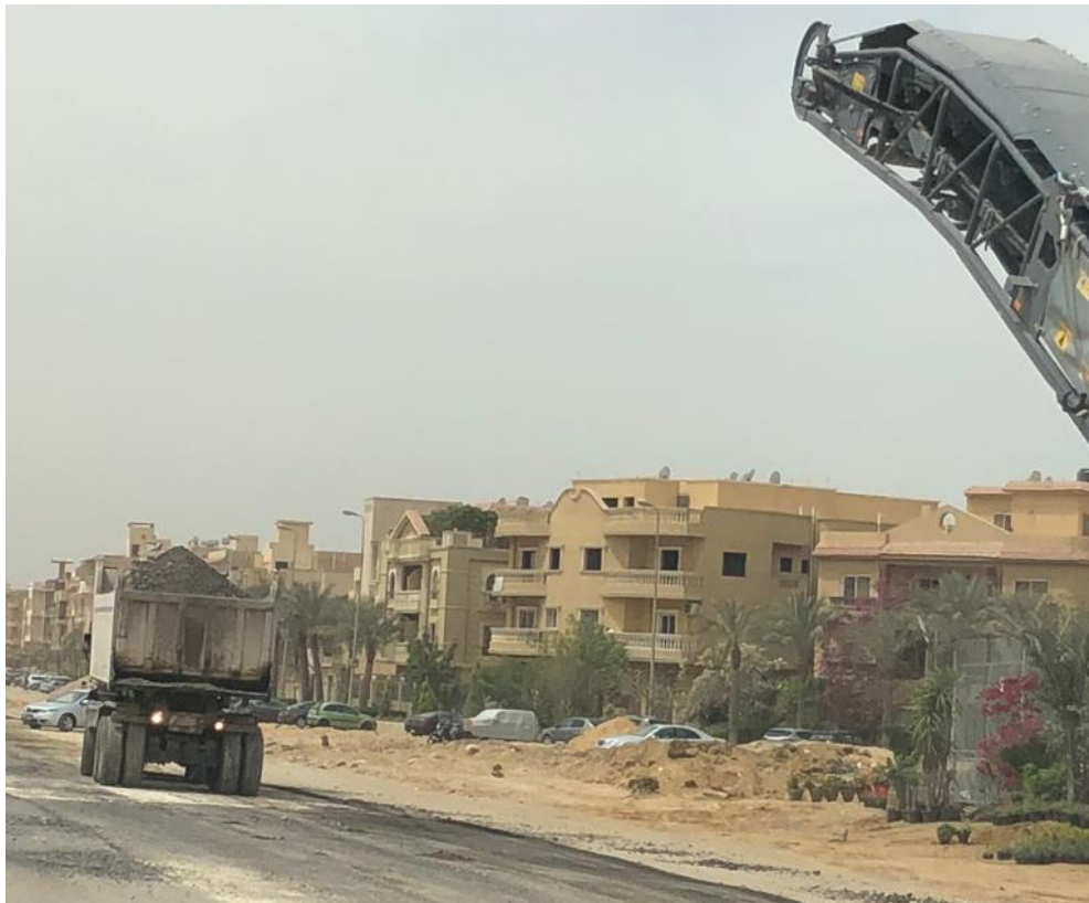
Figure 41: Road Works Machine and Truck on North 90 Street in April 2018
